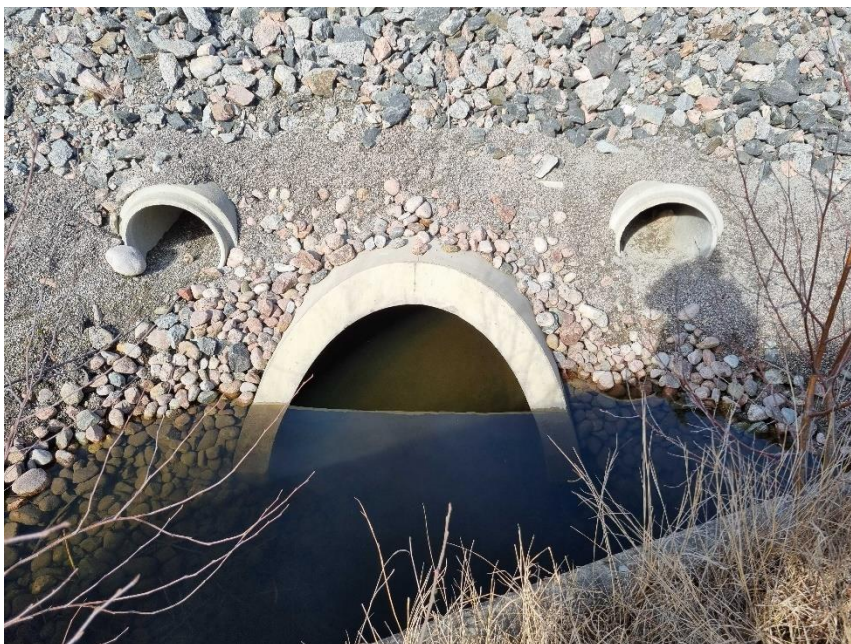
Figure 5 Picture of the ecoducts alongside the culvert at Ullnaån
