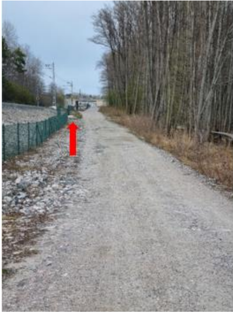
Figure 8 Picture of the position of the ecoduct at Täby prison
